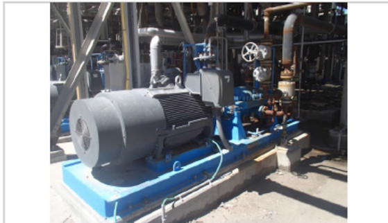
C1001020141 #2 Boiler Feed Water Pump (1-3)
